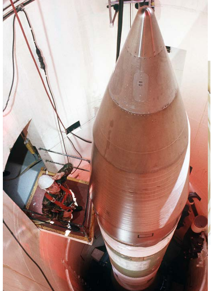
Missile maintenance crew members work on a Minuteman III ICBM in its silo. (Photo: U.S. Air Force)
