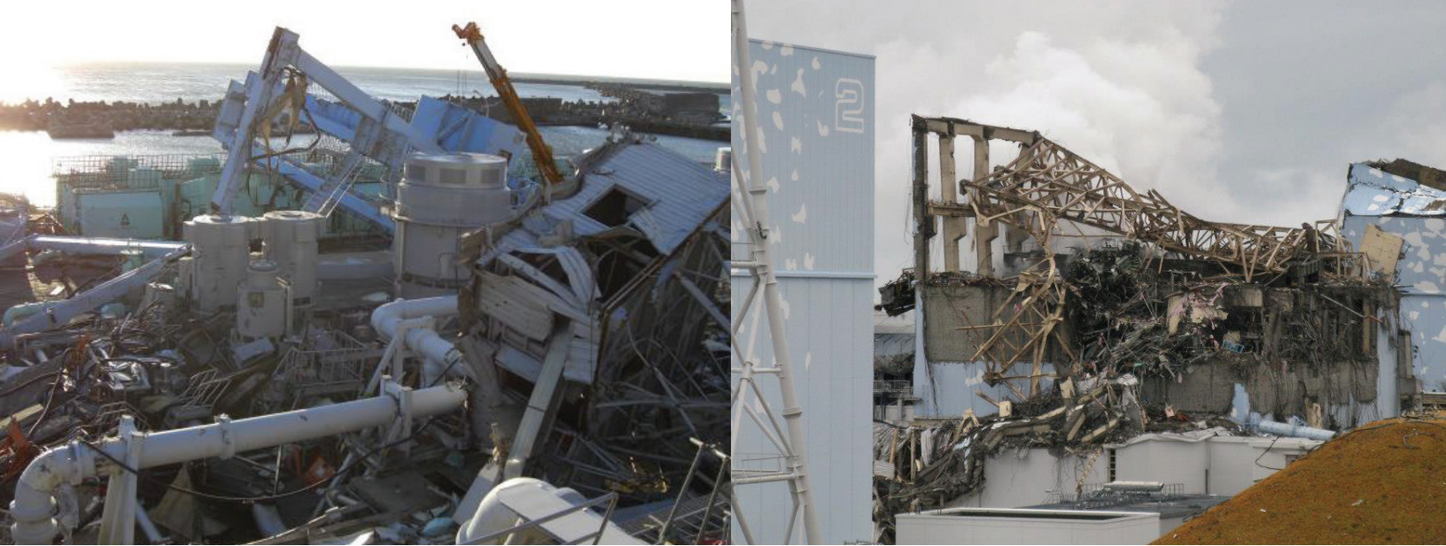
These photos showing the extensive damage at Fukushima were taken less than a week after the tsunami of March 11, 2011. Left: Conditions around Reactors 5 and 6. Right: The Reactor 3 building after an explosion blew off its upper floors. The explosion was triggered by the ignition of hydrogen gas created by reactor fuel overheating. Reactor buildings 1 and 4 suffered similar explosions in the days immediately following the tsunami. (Photos: TEPCO)
