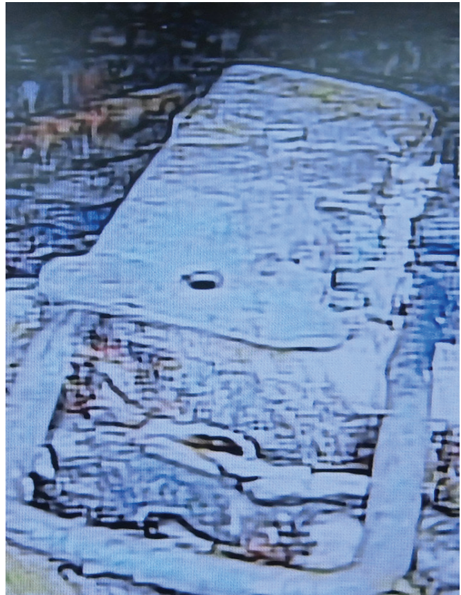
In April 2015, a small robot filmed the first images inside the PCV of Fukushima Reactor 1. Shown here are some of the debris it encountered inside the vessel. TEPCO reports that the robot recorded radiation levels of between 5 and 10 sieverts per hour (a tenth of what was expected) in some areas but levels as high as 25 sieverts per hour in others. A person receiving four sieverts in about one hour is at risk for death. (Photo: TEPCO)
